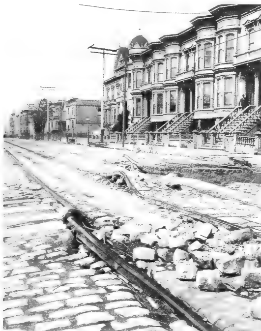
FIGURES 26–27. Figure 26 (left). Howard near 17th, San Francisco. Buckling of rails by compression. G.K. Gilbert photograph [GKG 2879], U.S. Geological Survey Photographic Archives, Denver, Colorado (also pl. 91 in Lawson [1908]). Figure 27 (right). Howard Street near 17th (East side of street). All houses shifted toward left. Tall house (center) dropped from its south foundation. G.K. Gilbert photograph [GKG 2893], U.S. Geological Survey Photographic Archives, Denver, Colorado.
